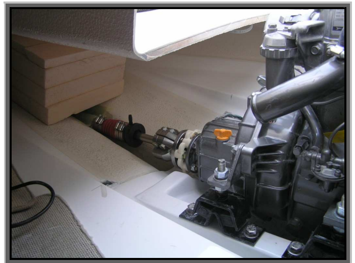
Above: The engine in its final position, fully bolted down and aligned on its custom moulding. This picture shows the engine coupling arrangement and water lubricated inner shaft seal (no need for grease lubrication or air bleeding after launching or drying out).
